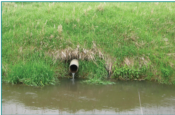
Drainage water management reduces the nitrate that flows to ditches and streams from tile drains compared to unmanaged drainage (shown above).
