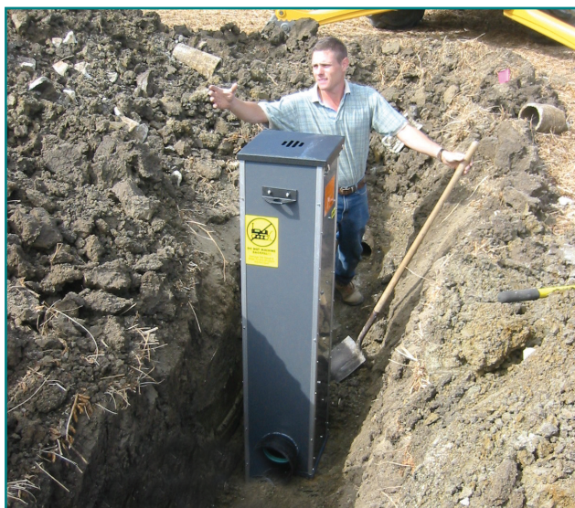
In drainage water management, water control structures are used to vary the depth of the drainage outlet. Flatter fields require fewer structures.
